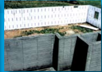
STEP 4: Once the concrete has cured and your forms are removed, the wall is ready for finish board application. Finish materials are easily installed by simply screwing into the exposed face of the ThermaEZE web for a secure hold. It's that easy! Supplemental foam adhesive may also be used for drywall installation.
