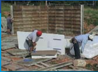
STEP 1: Insert ThermaEZE webs into the slots of the ThermaEZE insulation panel.
