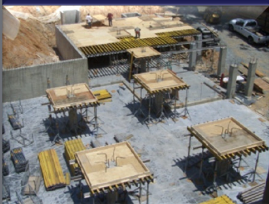
Formed Concrete Decks
